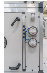
Fig 16: Magnehelic Gauge
